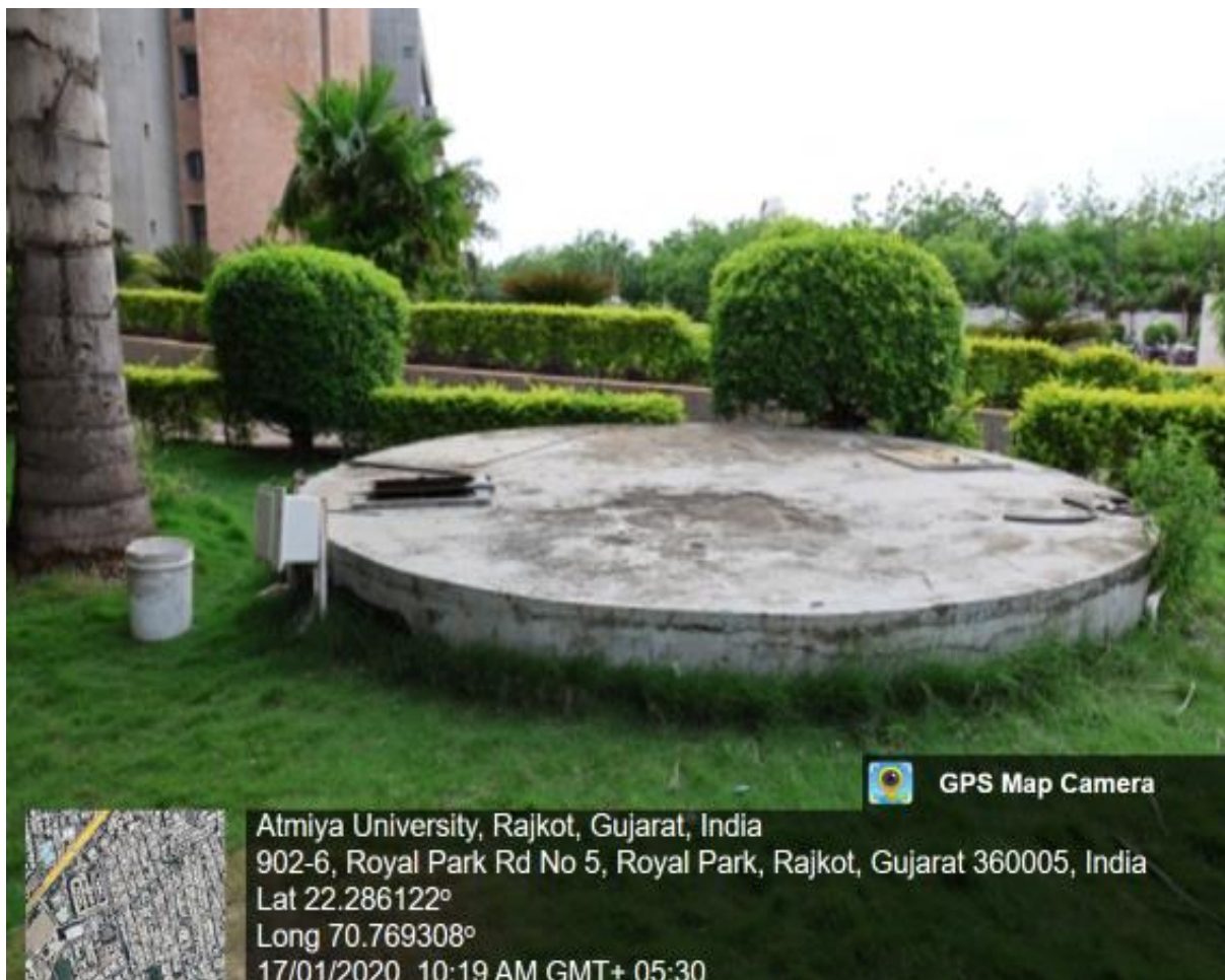
Rainwater Harvesting Tank
