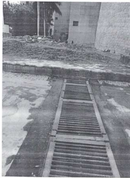
Rainwater Harvesting Tank
