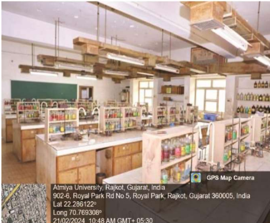
Acidic Fume Suction Panel
