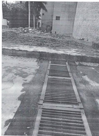
Rainwater Harvesting Tank
