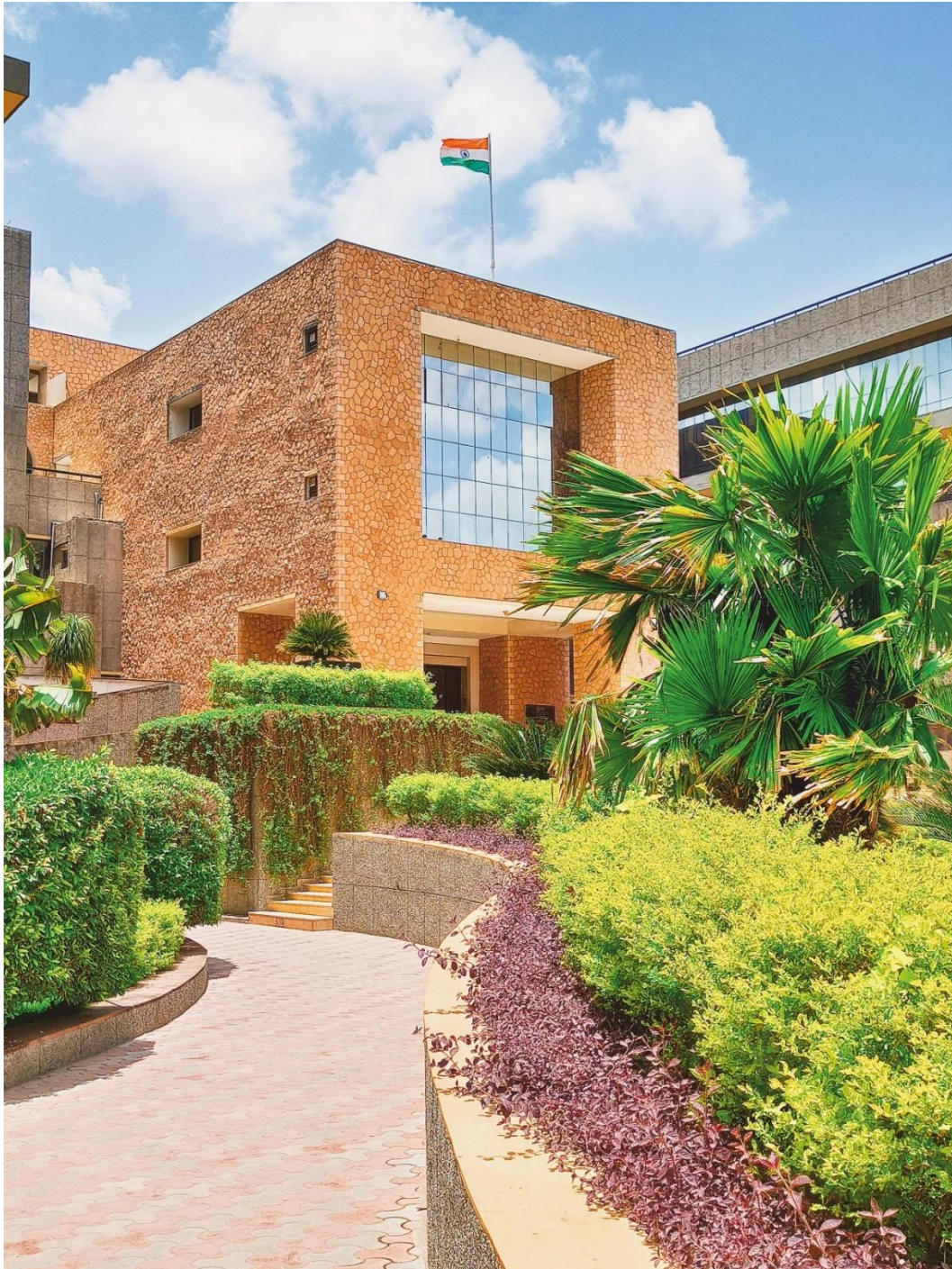
Insulating walls with natural shape stone fitting
