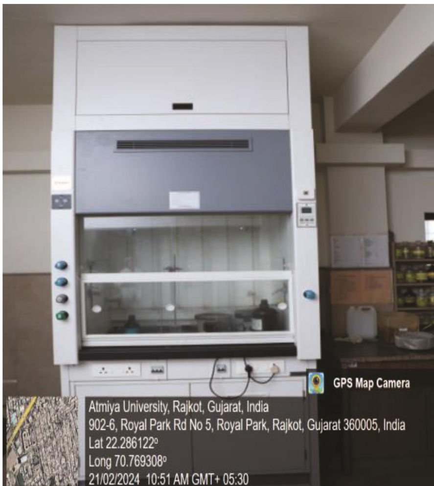
Fumehood at Chemistry Laboratory
