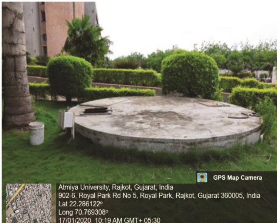
Rainwater Harvesting Tank
