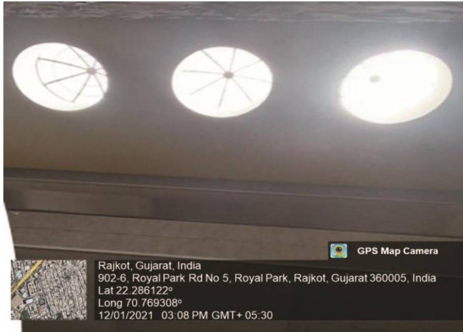
Natural Light and Ventilation in Academic Building
