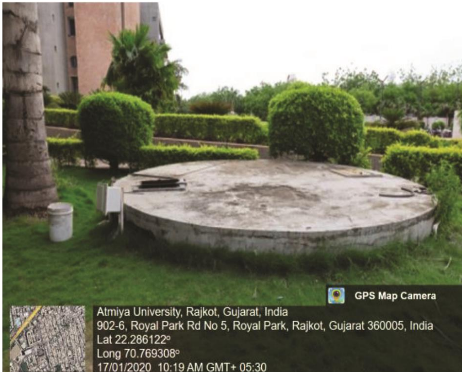
Rainwater Harvesting Tank
