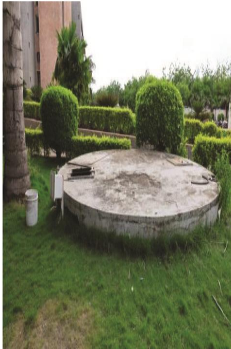
Rainwater Harvesting Tank
