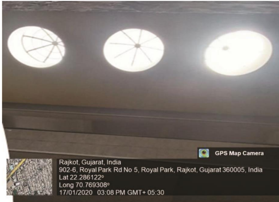
Natural Light and Ventilation in Academic Building
