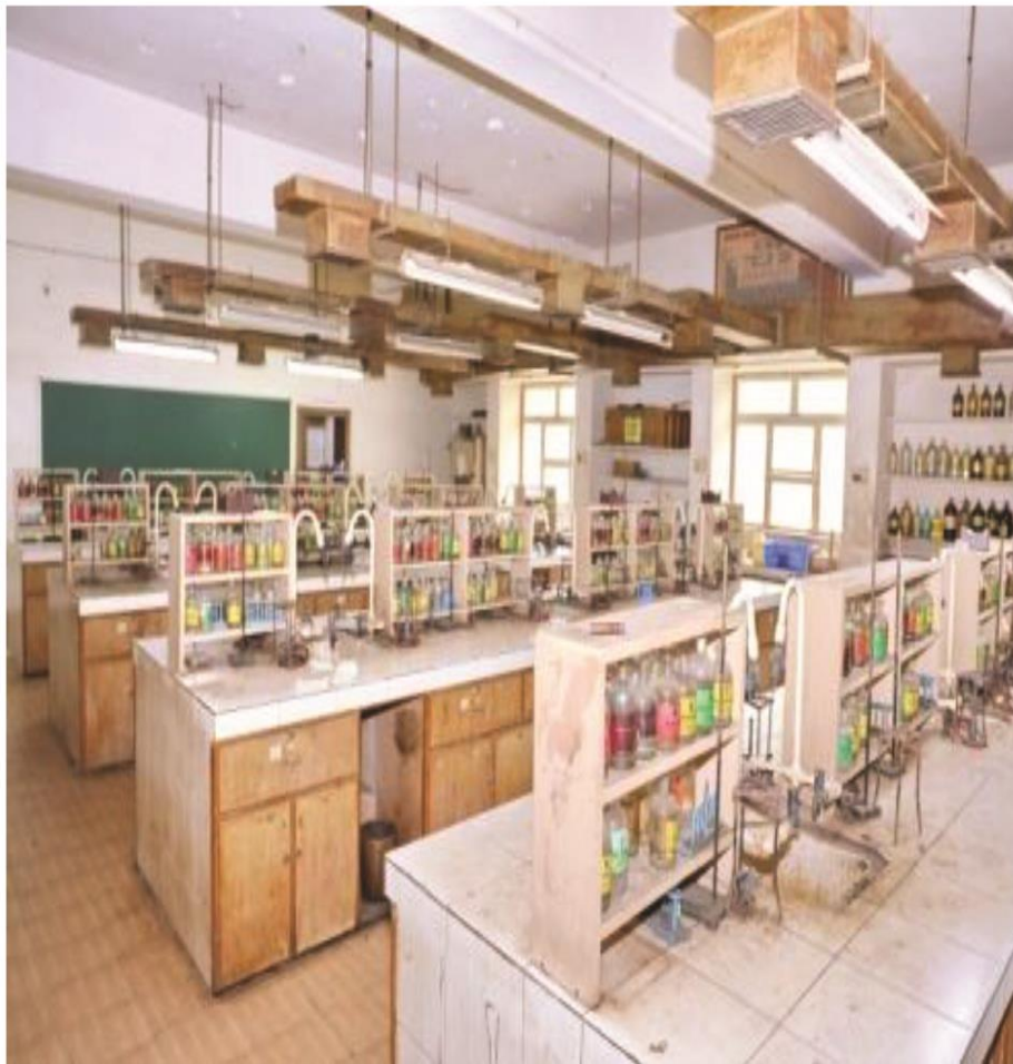
Acidic Fume Suction Panel
