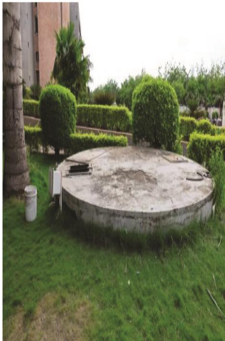
Rainwater Harvesting Tank
