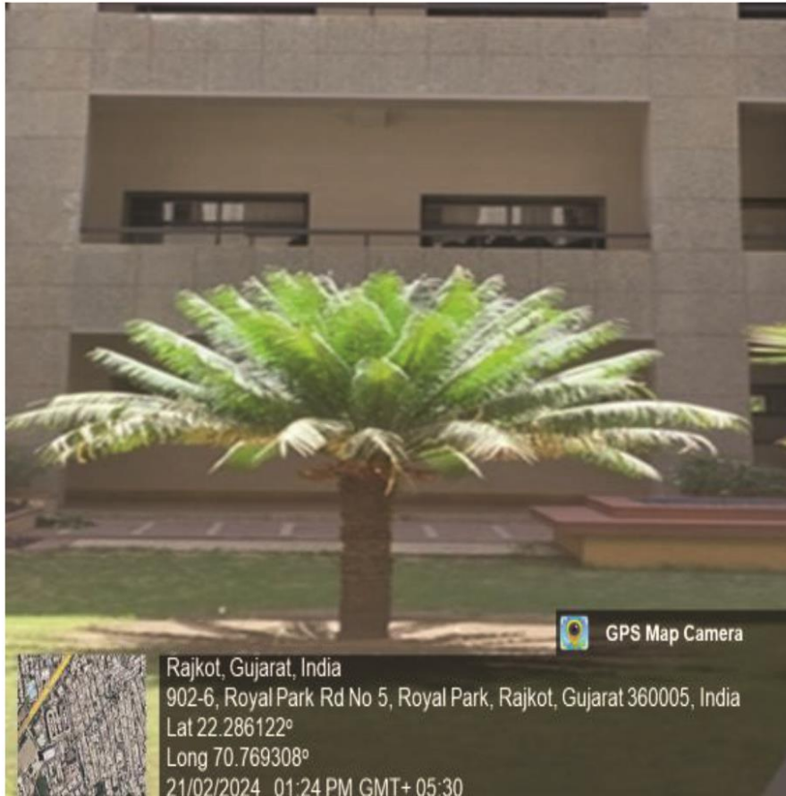
Natural Light and Ventilation in Academic Building
