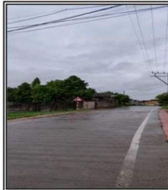
Cement Concrete Roads in the Village
